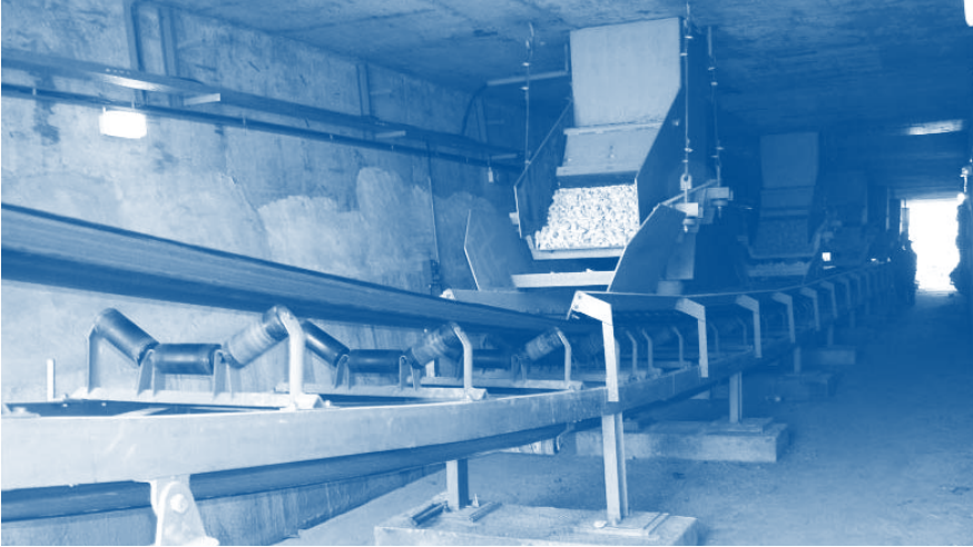
Transporting limestone to washing bay before sieving
