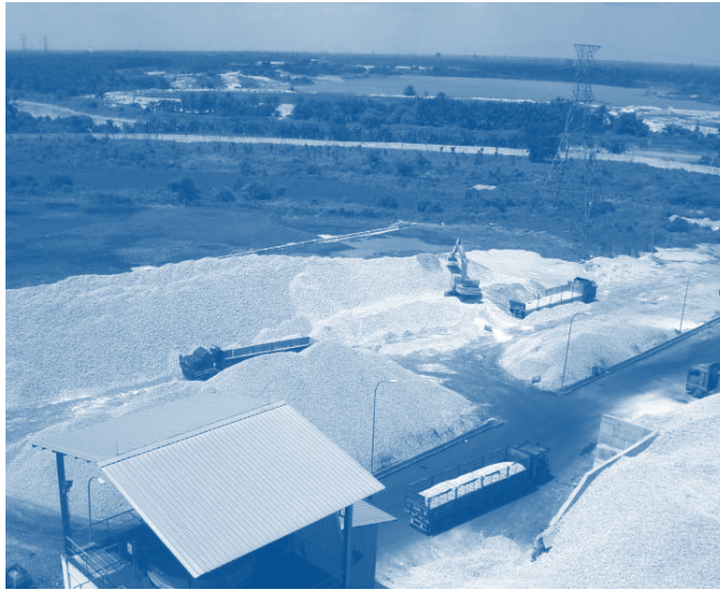
Limestone buffer storage yard
