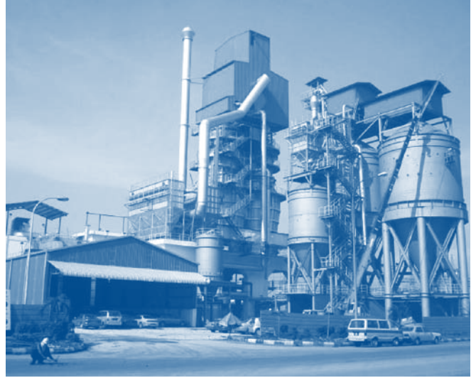
Limestone processing plant
