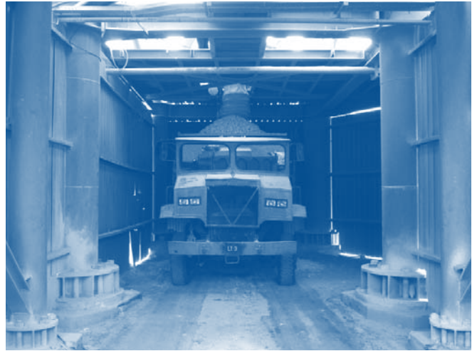
Quicklime unloaded from quicklime silo into truck
