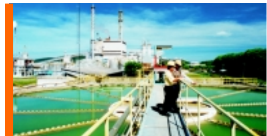
SFI water treatment plant. Loji rawatan air SFI.
