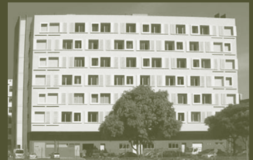
Newly renovated building at Arumugam road
