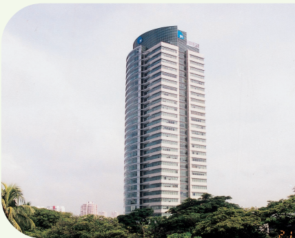
Angkasa Building Materials supplied fabricated steel reinforcement bars for JTC Headquarter
