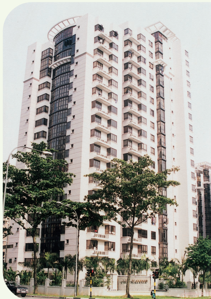
Angkasa Building Materials supplied steel for the construction of The Mayfair condominium
