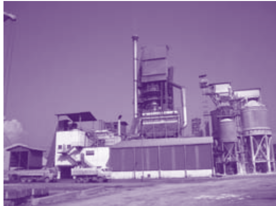
Quicklime Production Plant - Phase 1
