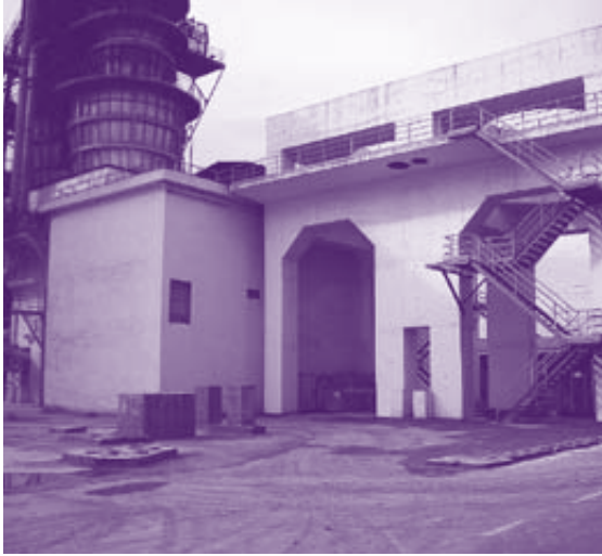
Quicklime Production Plant - Phase 2 (construction in progress)
