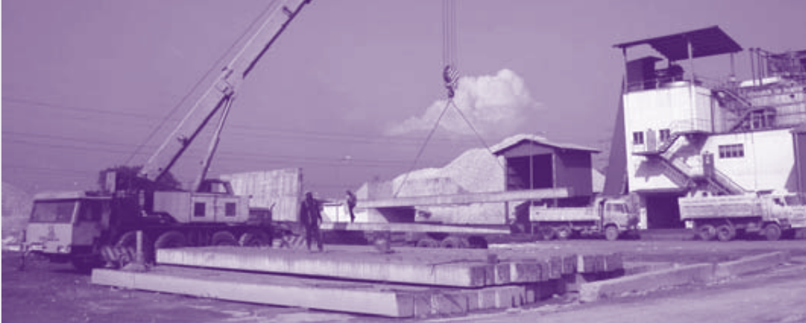
Hydrated Lime Production Plant (construction in progress)
