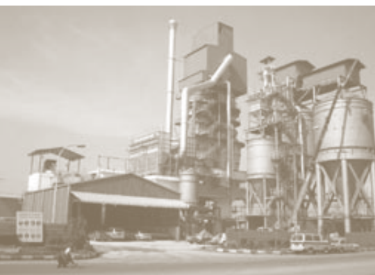
Limestone processing plant
