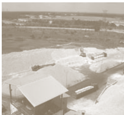
Limestone buffer storage yard
