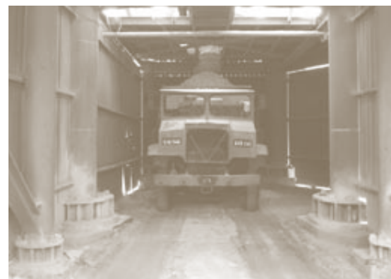
Quicklime unloaded from quicklime silo into truck
