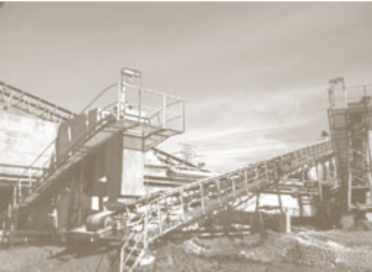
Limestone diverted to double deck washing screen after the tunnel
