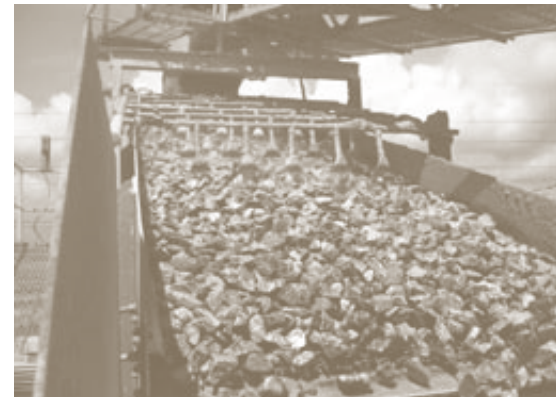
Water nozzles spray water over kiln stone remained on upper screen
