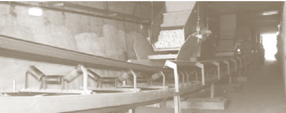
Transporting limestone to washing bay before sieving
